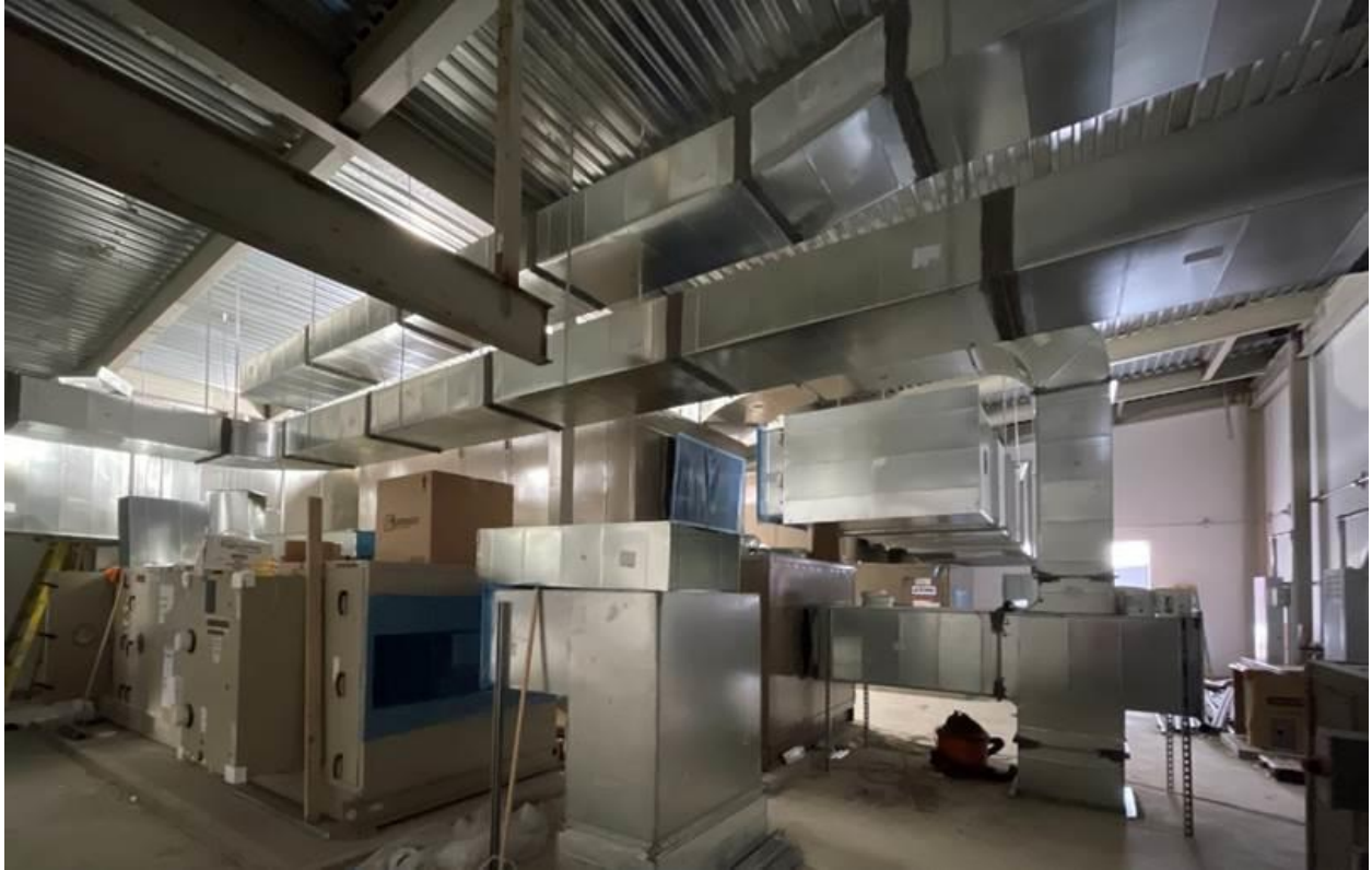
Ductwork and ventilation equipment in the mechanical room over the locker rooms
