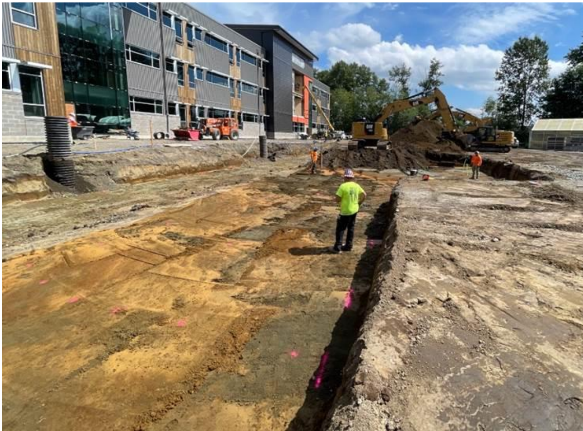
Excavating for the underground stormwater storage system on the Academic Wing's south side
