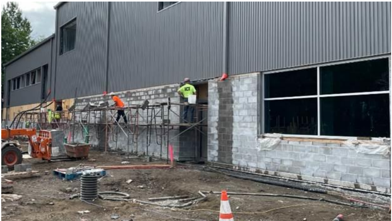
Masonry blocks being installed at the north side of the locker room area
