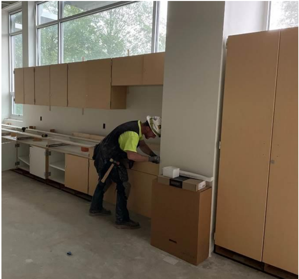
Cabinet installation on the Academic Wing's second floor
