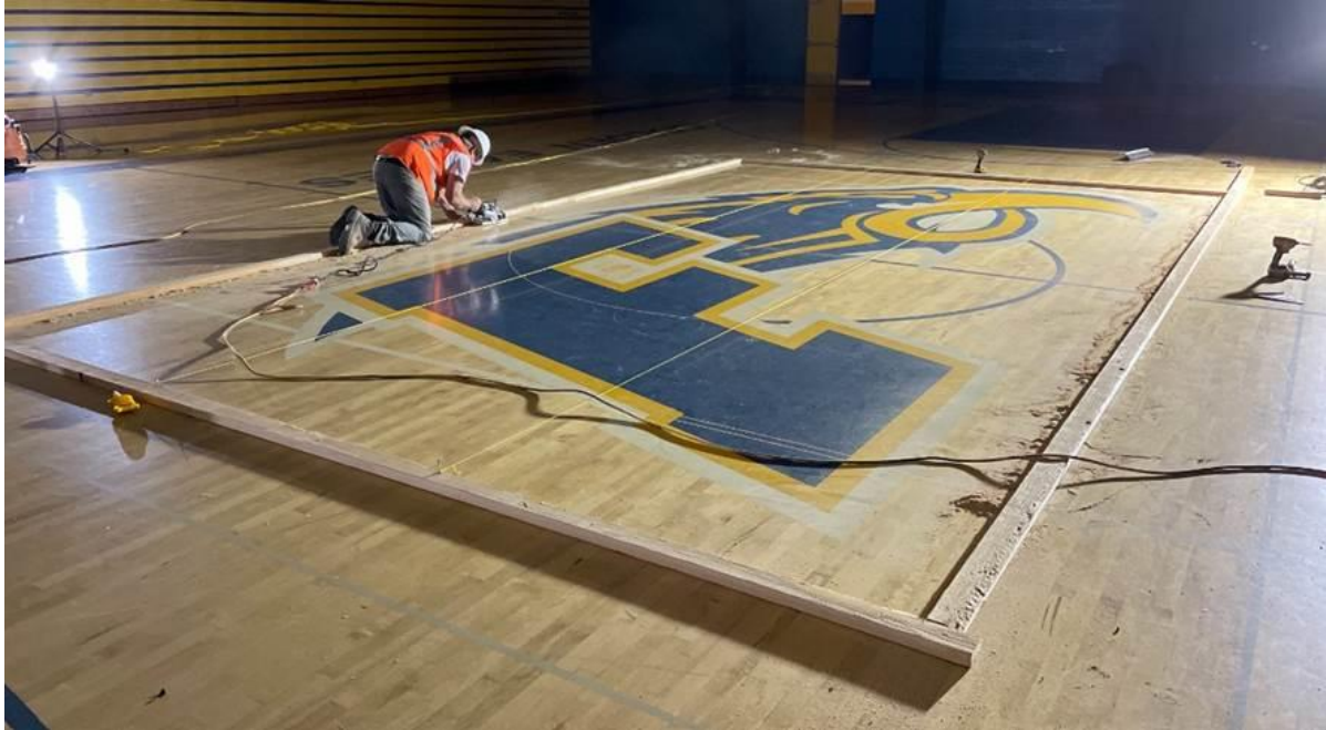
Old Gymnasium flooring being salvaged for reuse
