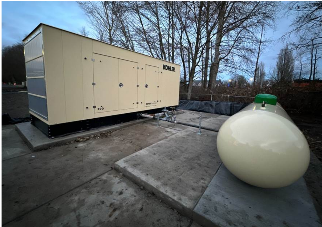
The emergency generator is in place and connected to the backup propane fuel supply
