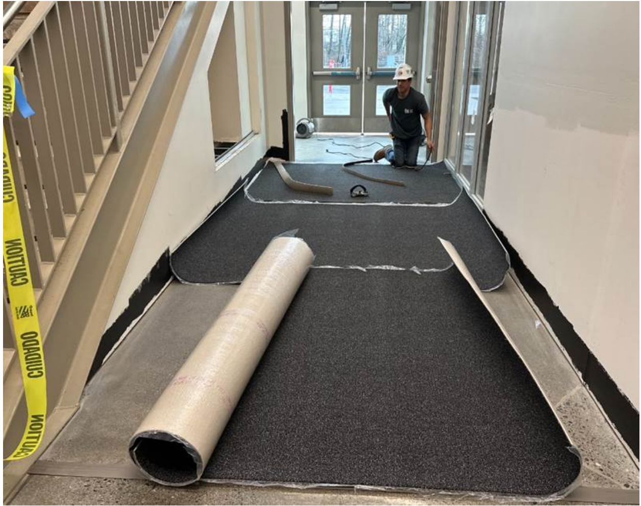
Walk-off carpet installation at the eastern Academic Wing stairwell
