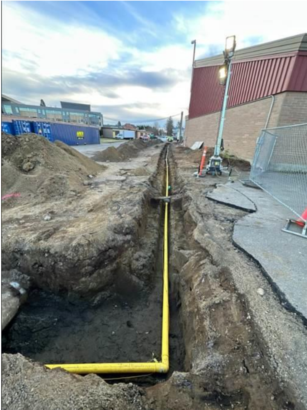
Natural gas installation adjacent to the Performing Arts Center
