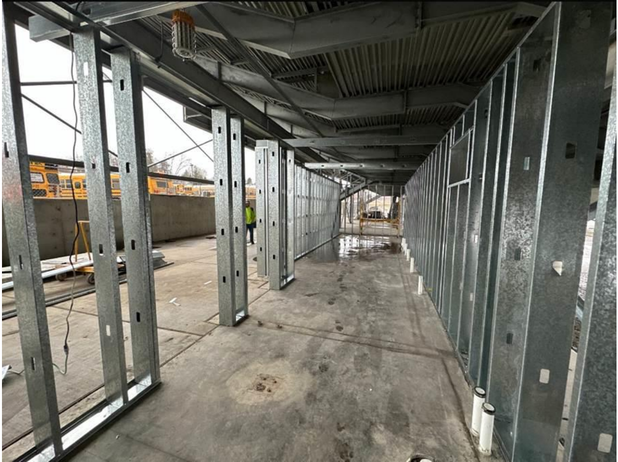
Framing of the football field grandstand restrooms and concessions area
