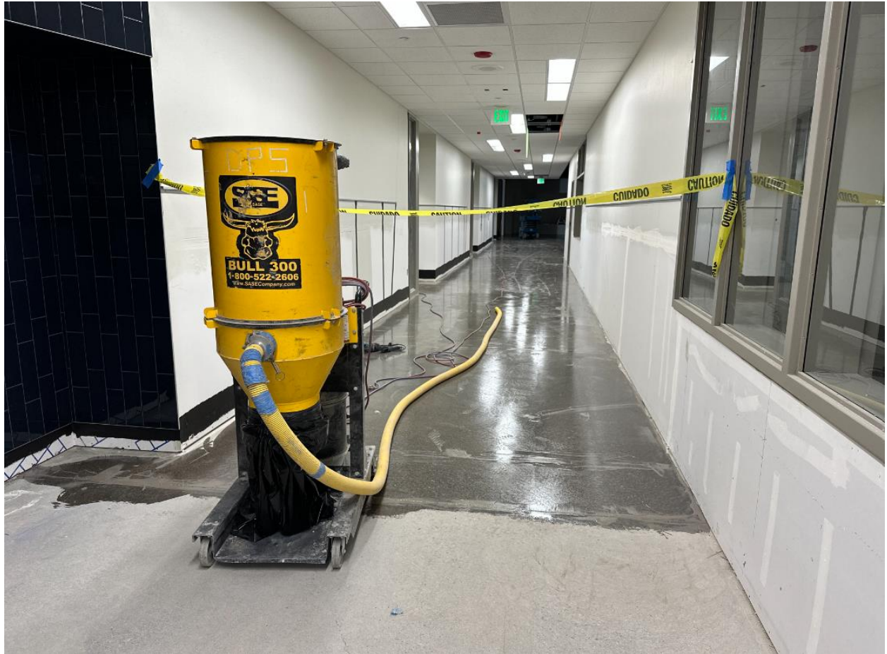
Grinding and polishing of concrete corridor floors in the Academic Wing
