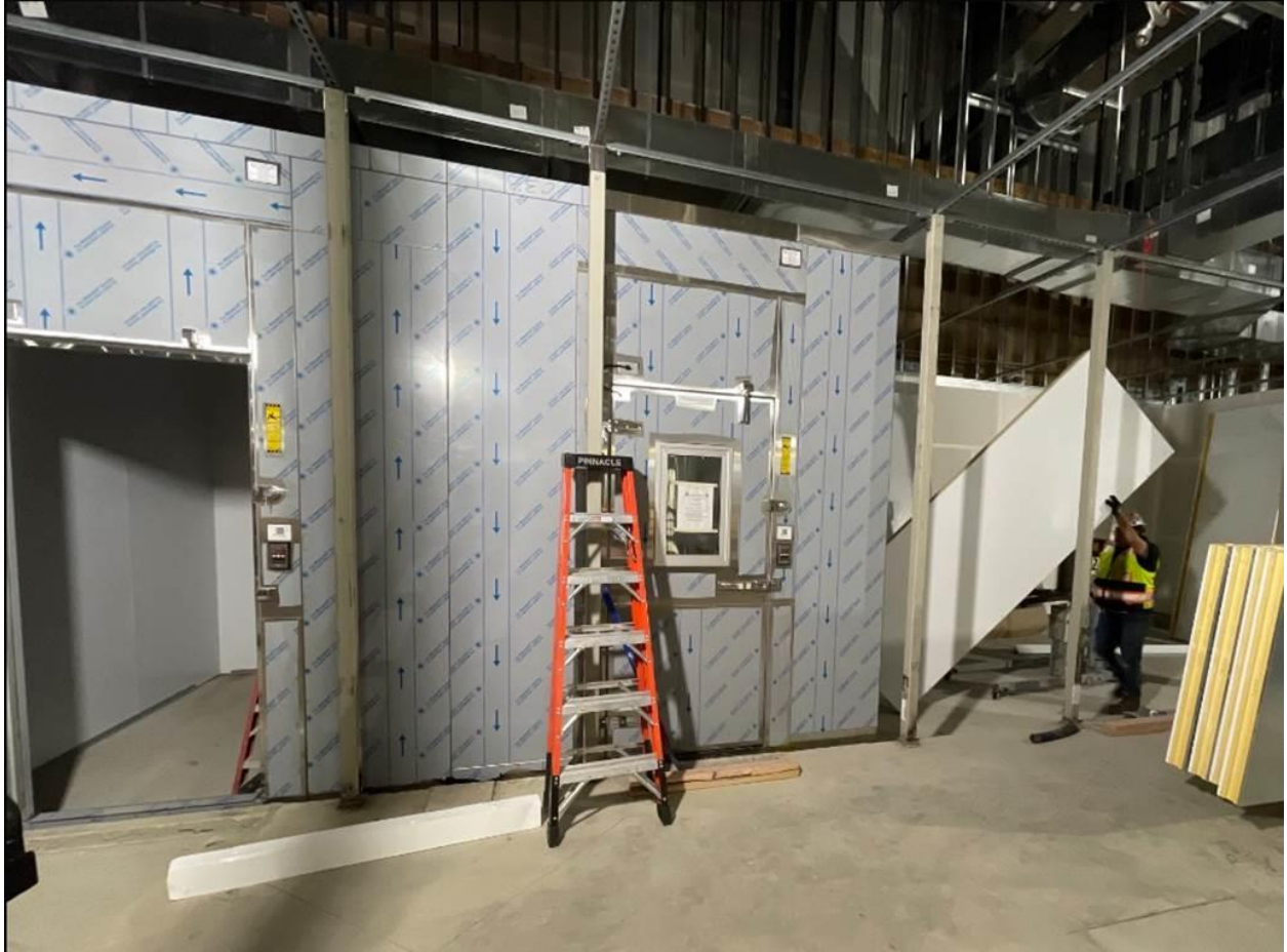
Walk-in cooler installation in the Kitchen Area
