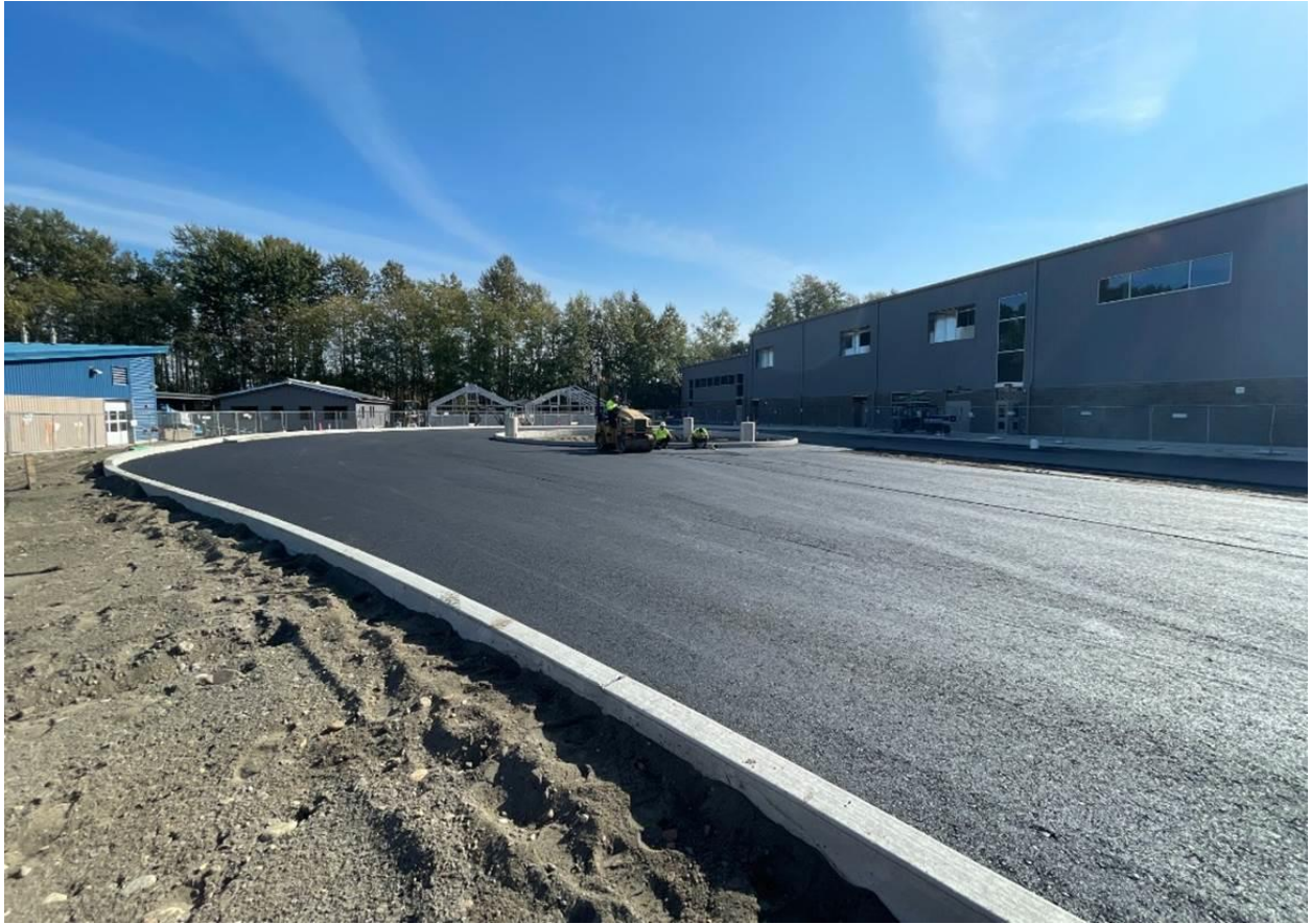
Asphalt being laid in the new bus loop north of the new gym
