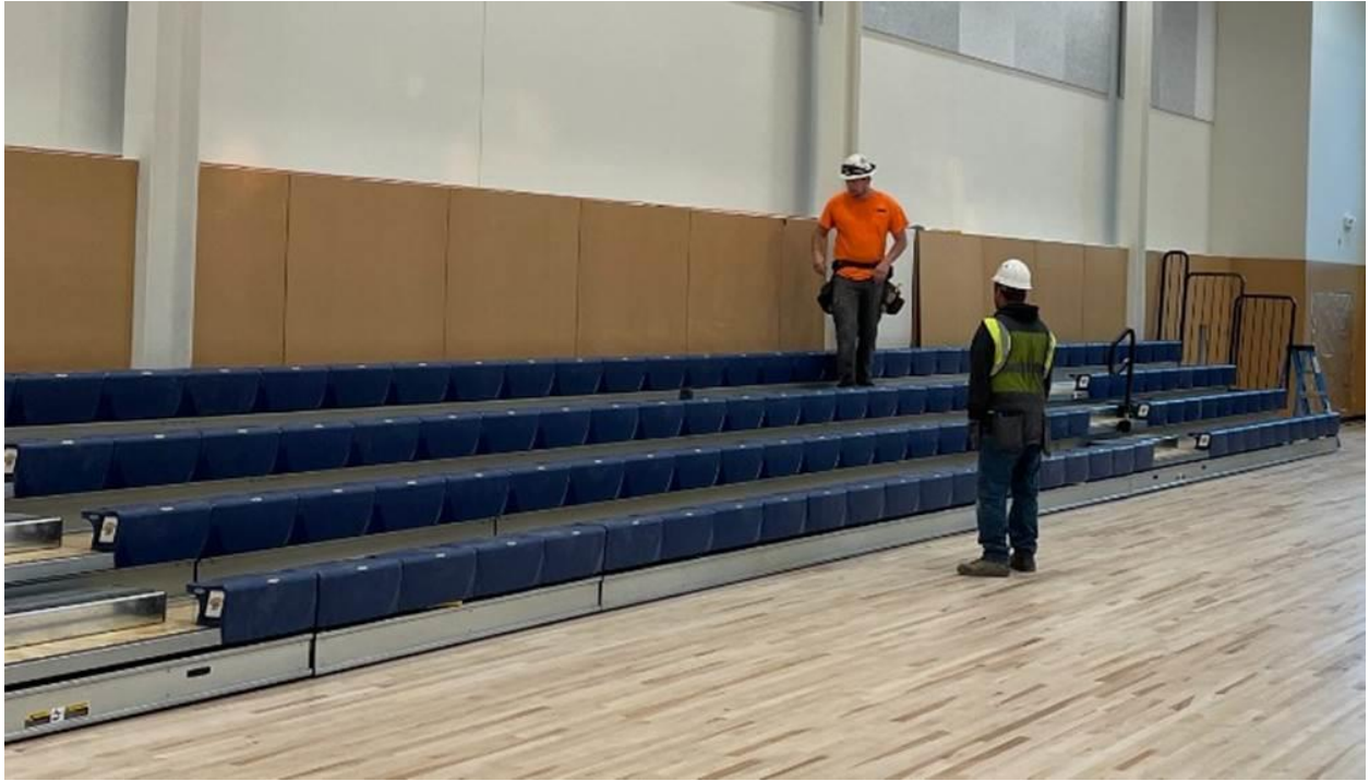
Bleacher installation in the Auxiliary Gym
