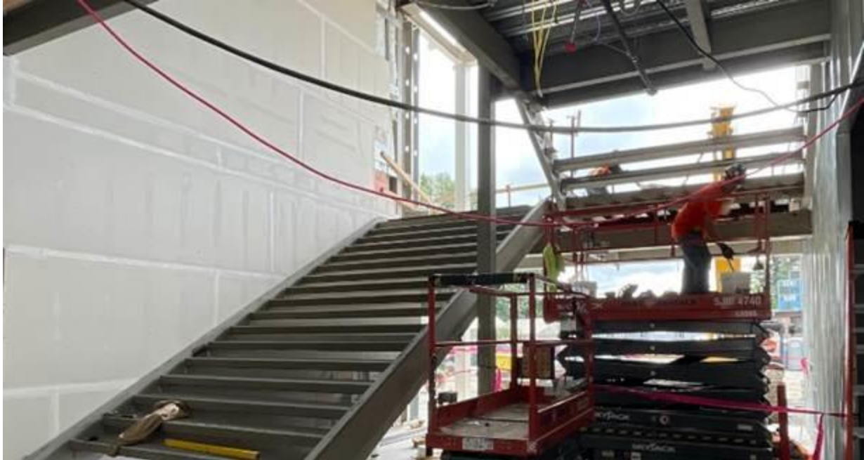
Last set of stairs receiving the precast treads
