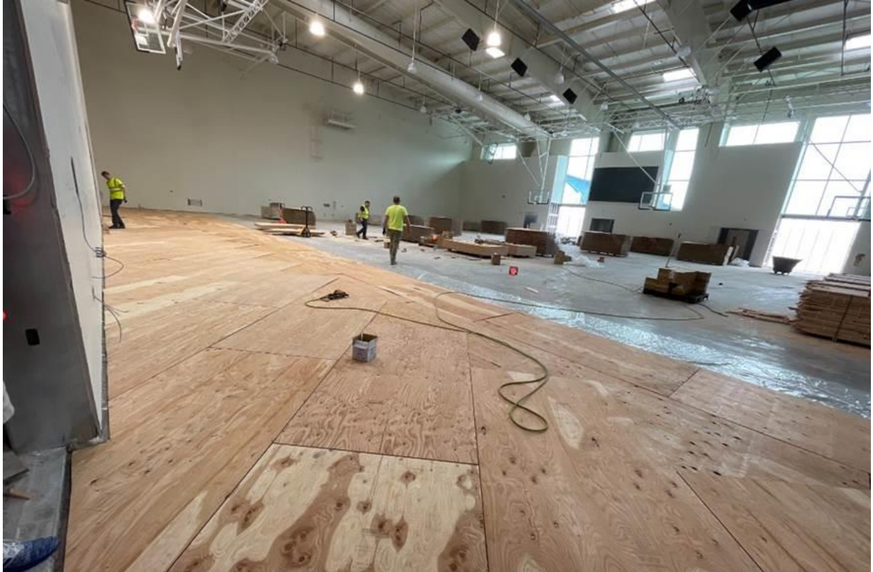
Wood flooring system being installed in the Main Gym
